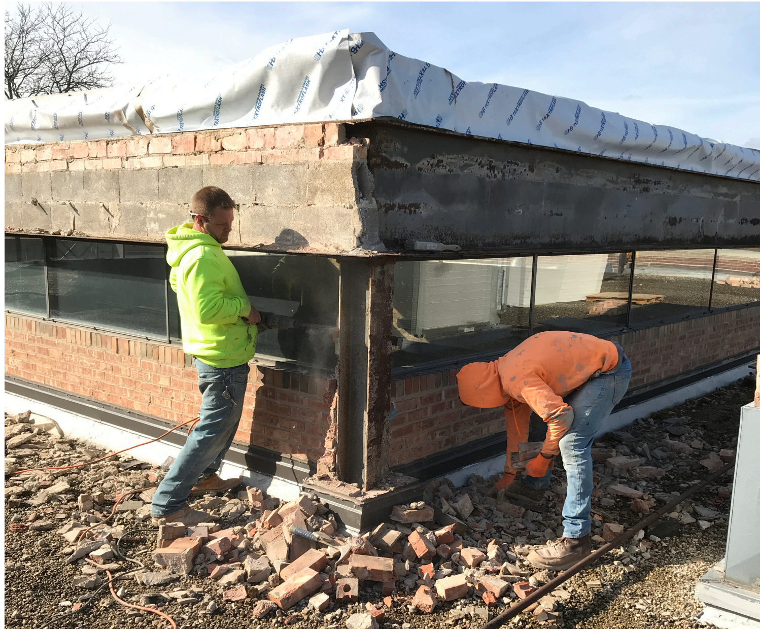
Clerestory Repair in Progress
