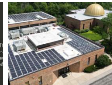
SOLAR ENERGY PANELS
