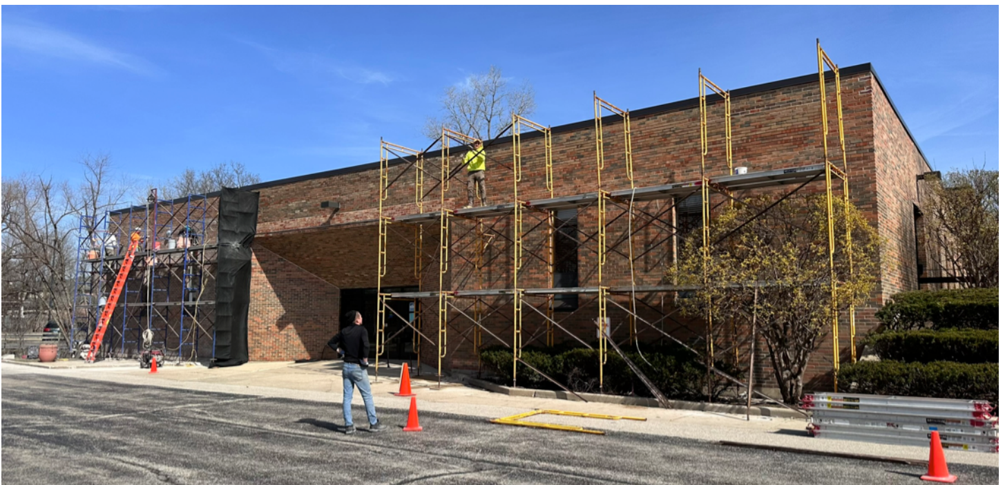
Brick Tuck Pointing project on Community Center Spring 2024
