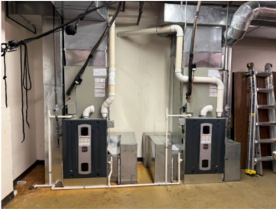
The replacement of the HVAC systems serving the rooms under the gym have been replaced. Note that the a/c condensers have been removed from the Agape playground.
