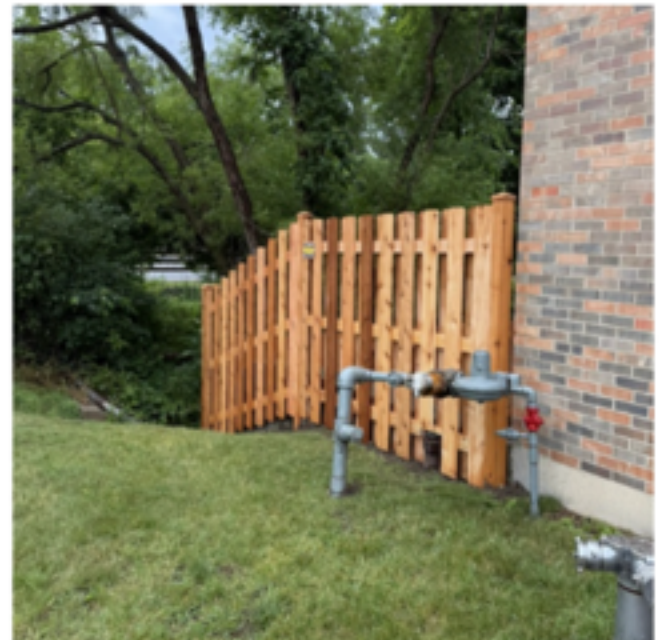
The four-foot open fence surrounding the Agape playground has been replaced with a new six-foot board on board cedar fence.
