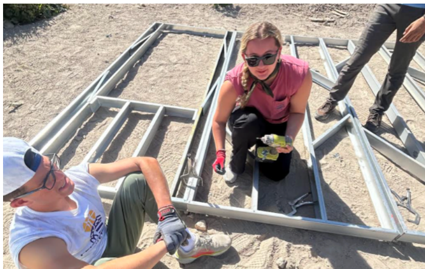
Mia Dehnert and Yianni Papadopoulos drilling in the beams to the home 7/30/26
